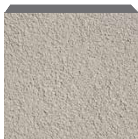
Healthy painted substrate (no cracks and flaking)
